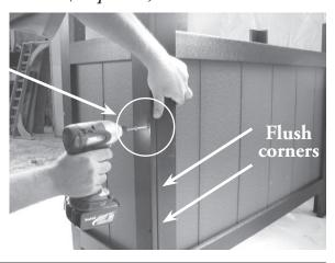
**Step #2** With the shorter overhang situated above the shelve opening, place bar top on the side uprights. Then fasten all sides using <sup>3</sup>/<sub>4</sub>" screws.
